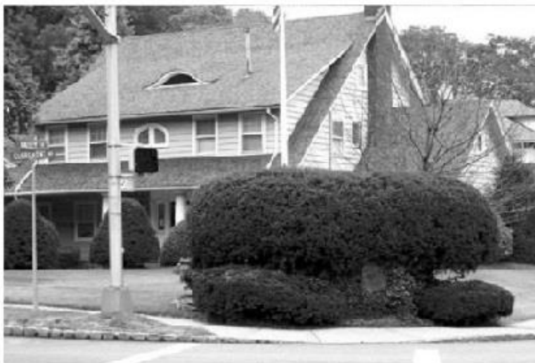
2. Washington HQ (Crane House, Montclair, NJ)
