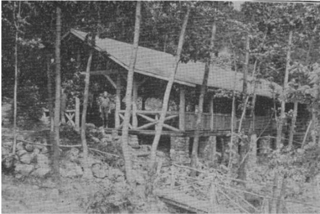
1. Original Mess Hall <1961
