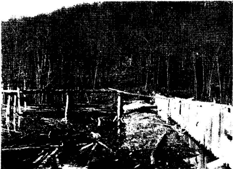
Building the Core Wall of the Dam
